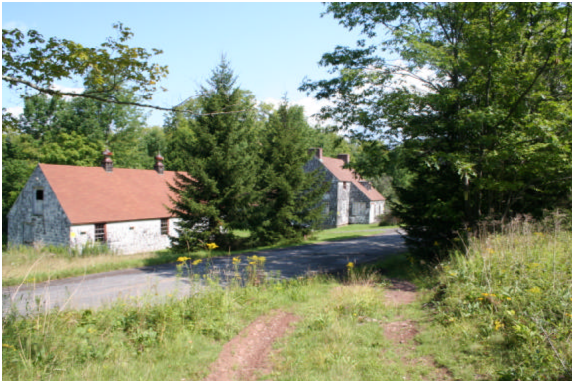
Photo 66. View of field entrance to the northern end of the northern APE area, facing northeast.
