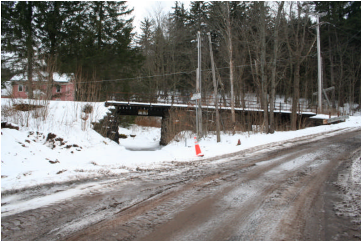
Photo 16. View of railroad bridge crossing Fleischmanns Heights Road and Depitts Lane, facing southwest.
