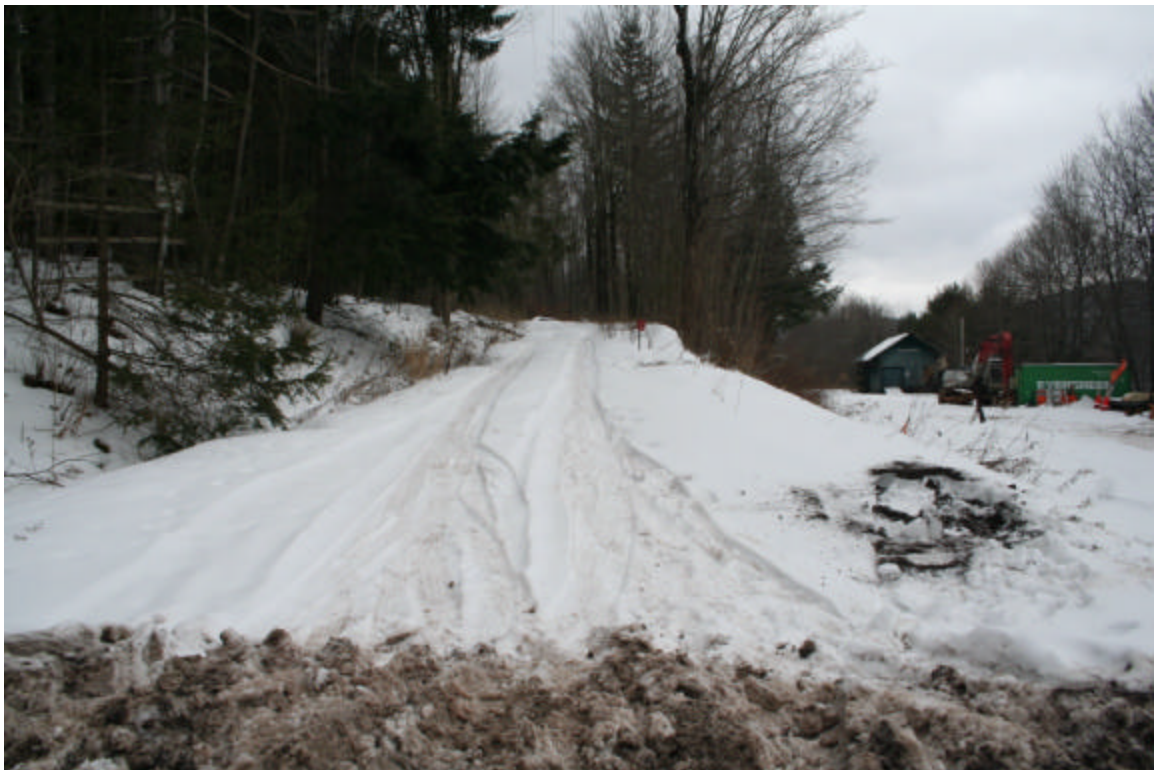
Photo 12. View from the intersection of the K-Wells access road and Fleischmanns Heights Road, facing west.
