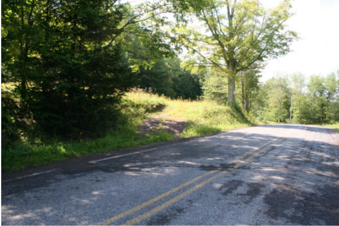
Photo 67. View of field entrance to the northern APE area from NYS Route 44A, facing southwest.
