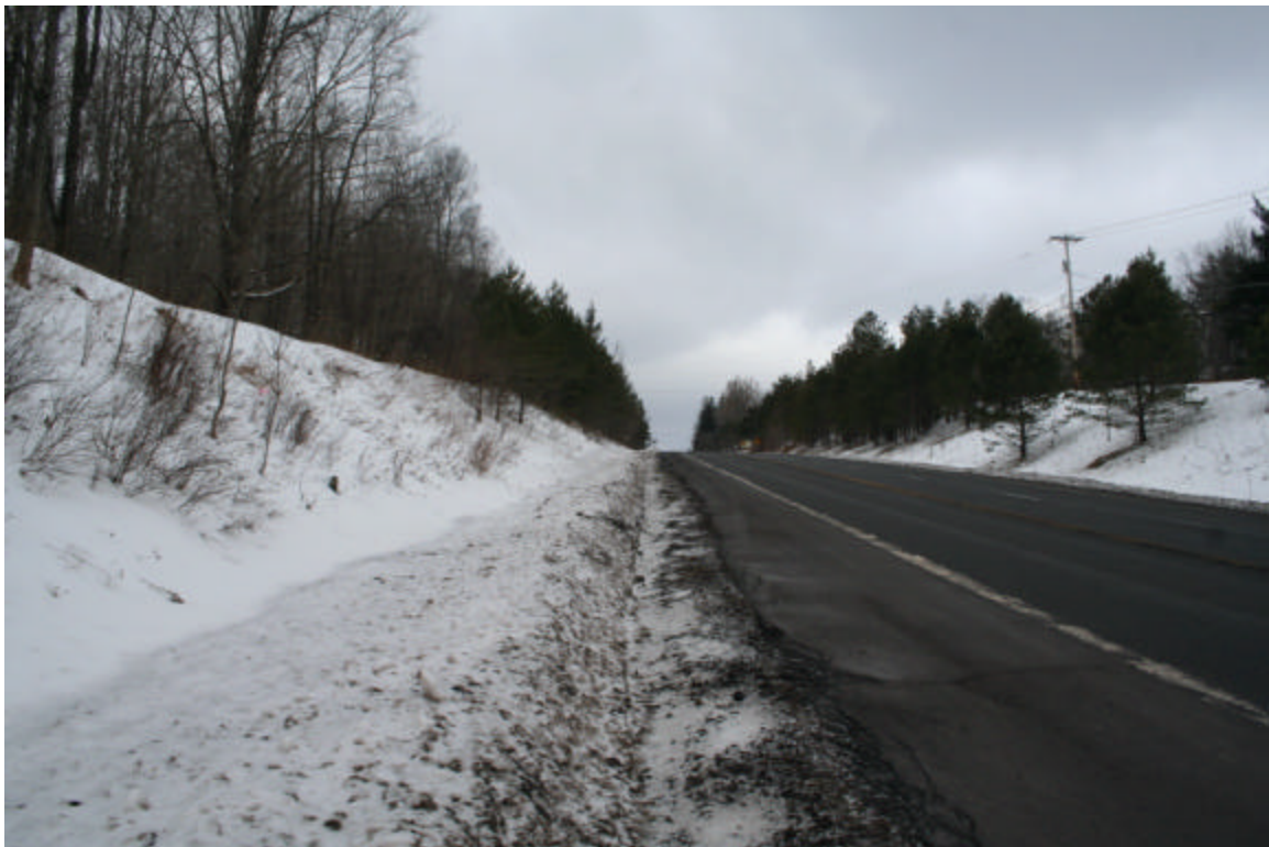
Photo 66. View along the proposed sewer main route on the south side of NYS Route 28, facing northwest.
