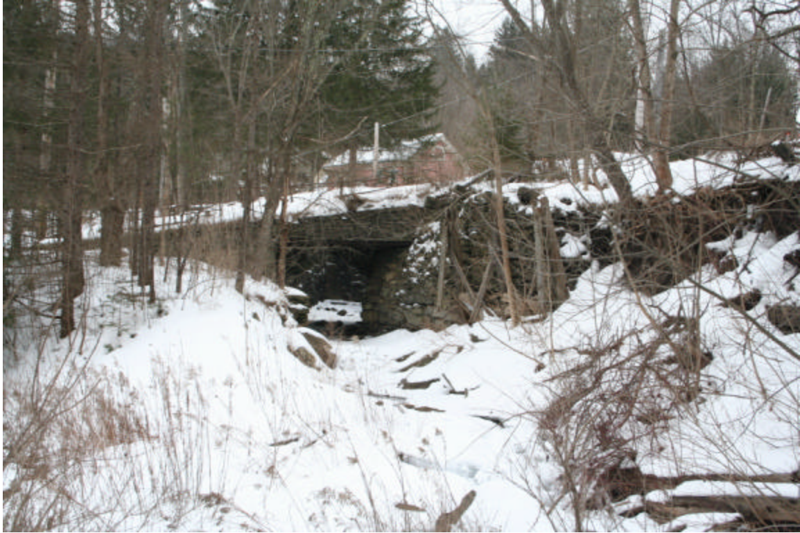
Photo 17. View of stone culvert under Fleischmanns Heights Road, facing southeast.
