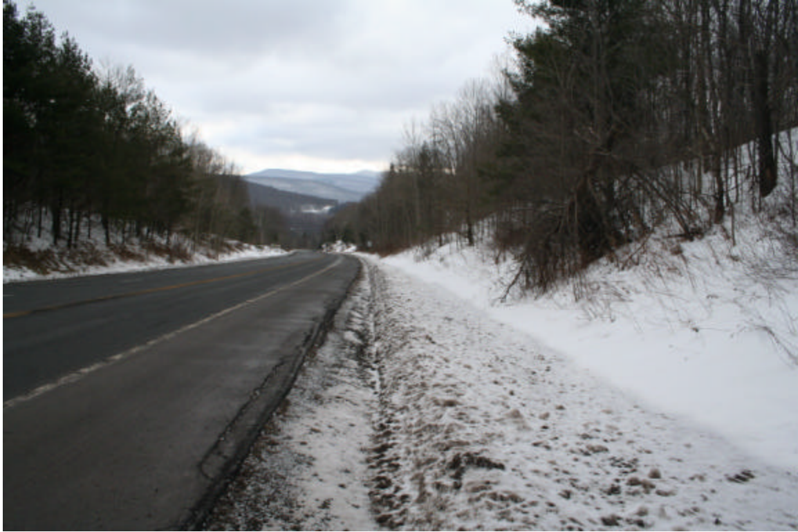
Photo 67. View along the proposed sewer main route on the south side of NYS Route 28, facing southeast.
