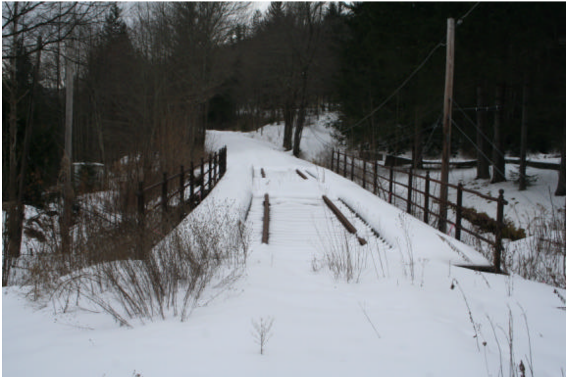
Photo 14. View of railroad bridge crossing Fleischmanns Heights Road and Depitts Lane, facing east.
