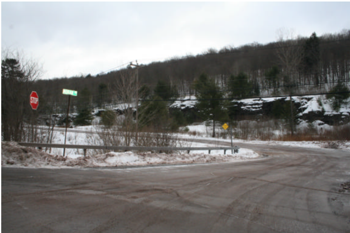
Photo 44. View of the water main route from the intersection of NYS Route 28 and Moran Road, facing south.
