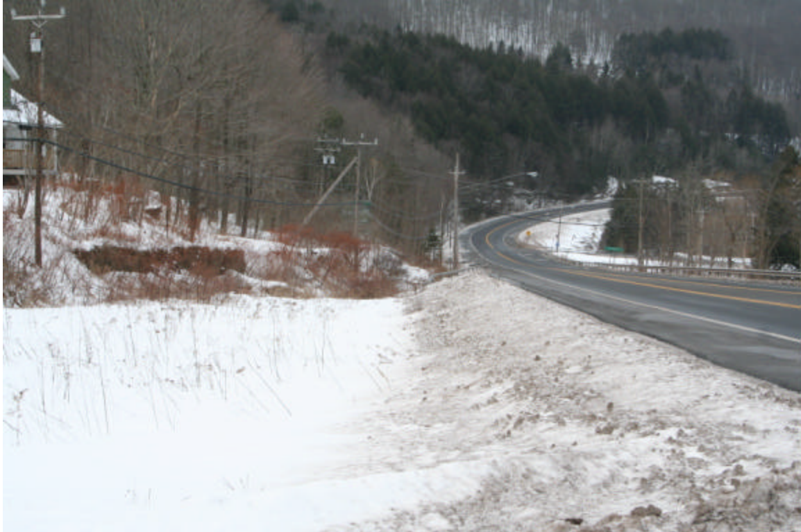
Photo 43. View of the water main route from the intersection of NYS Route 28 and Moran Road, facing west.
