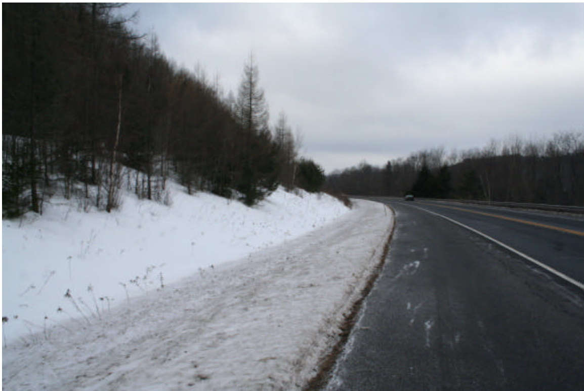
Photo 36. View along the proposed water main route on the south side of NYS Route 28, facing northwest.
