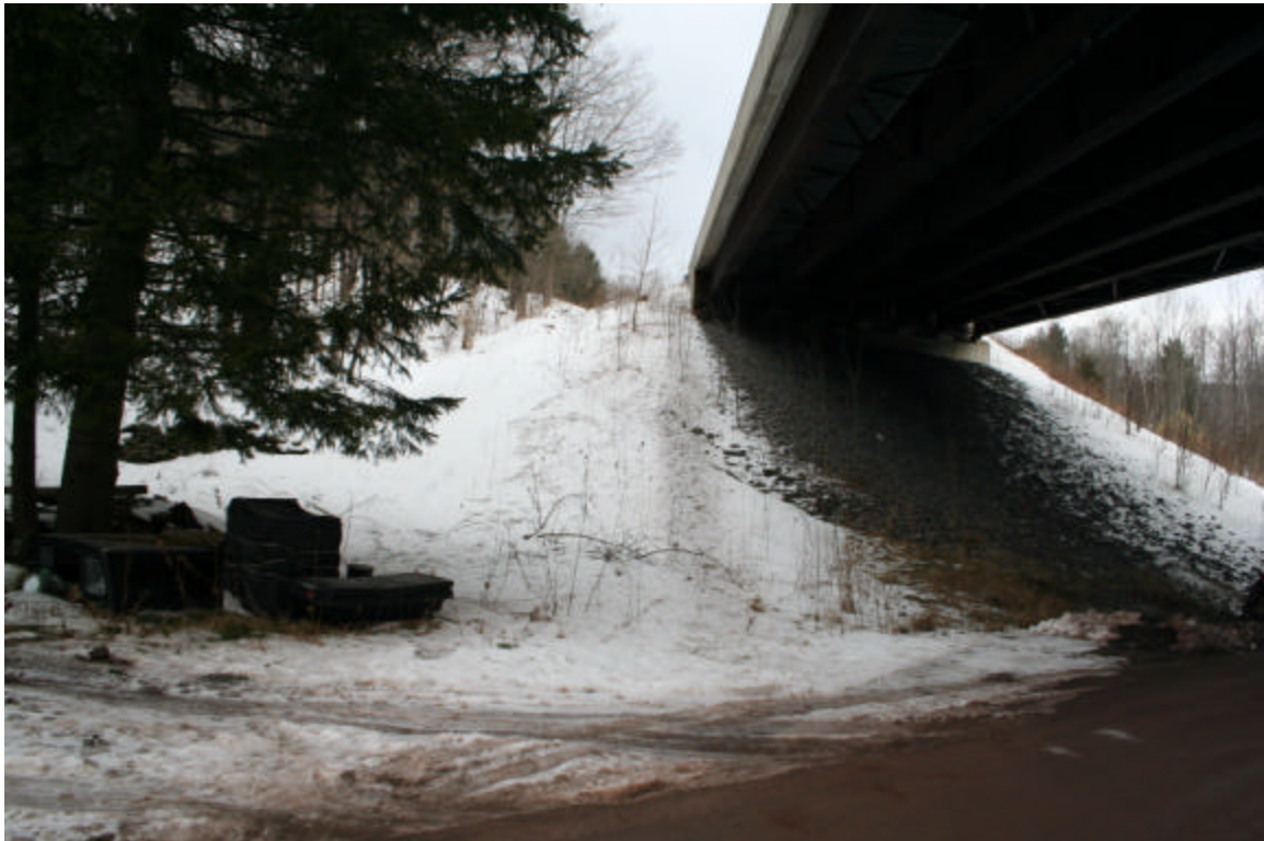
Photo 74. Portion of panoramic view from the east end of the proposed sewer main route, facing northwest.
