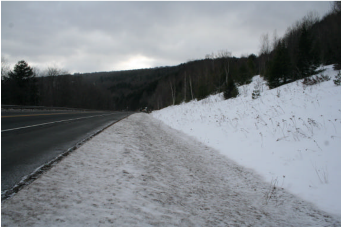
Photo 37. View along the proposed water main route on the south side of NYS Route 28, facing southeast.
