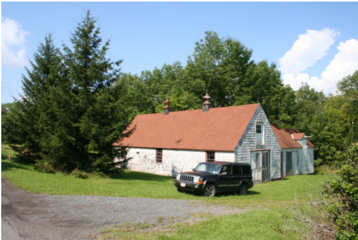
Photo 70. View of barn on the north side of NYS Route 44A, facing northwest.
