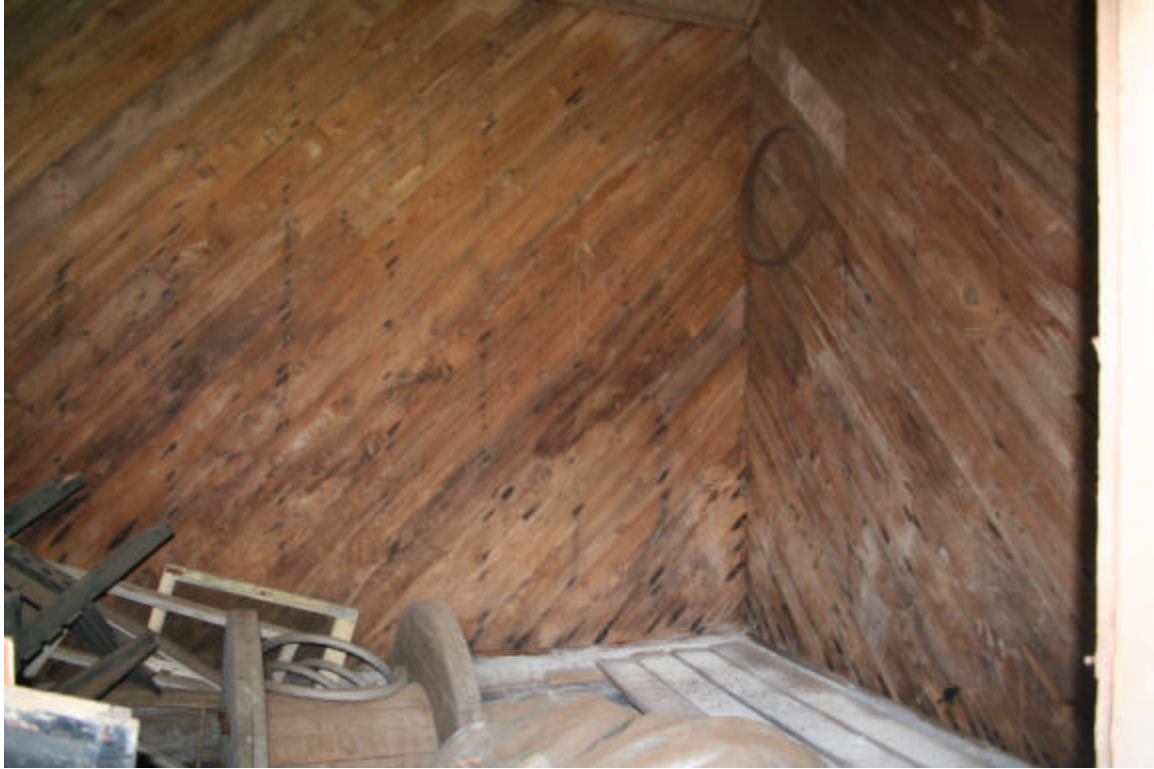
Photo 73. Interior of ice house at the farm complex on the north side of NYS Route 44A, facing southwest.
