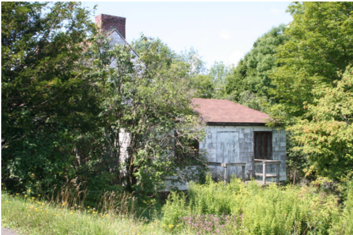
Photo 78. View of historic farm house on the north side of NYS Route 44A, facing west.
