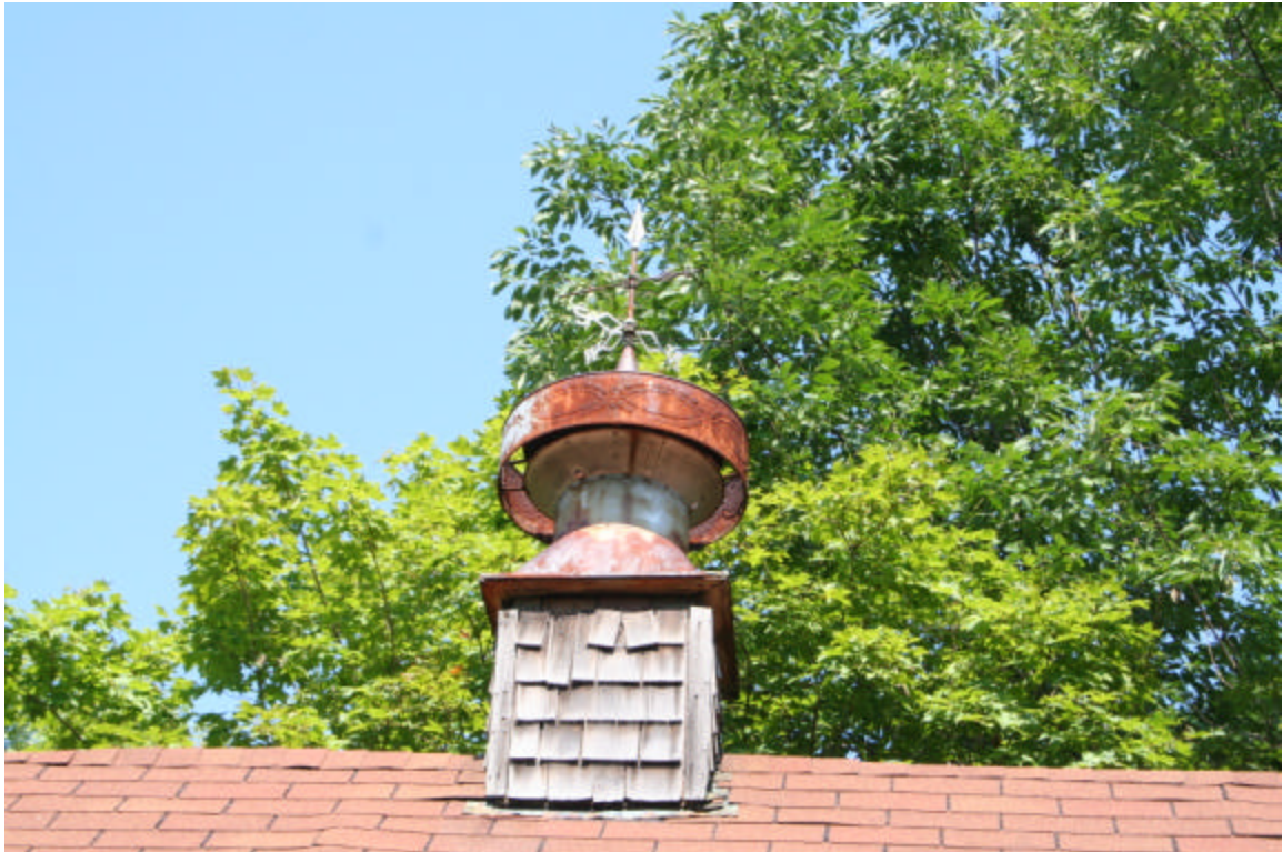
Photo 77. View of decorative ventilator on the barn located on the north side of NYS Route 44A, facing north.
