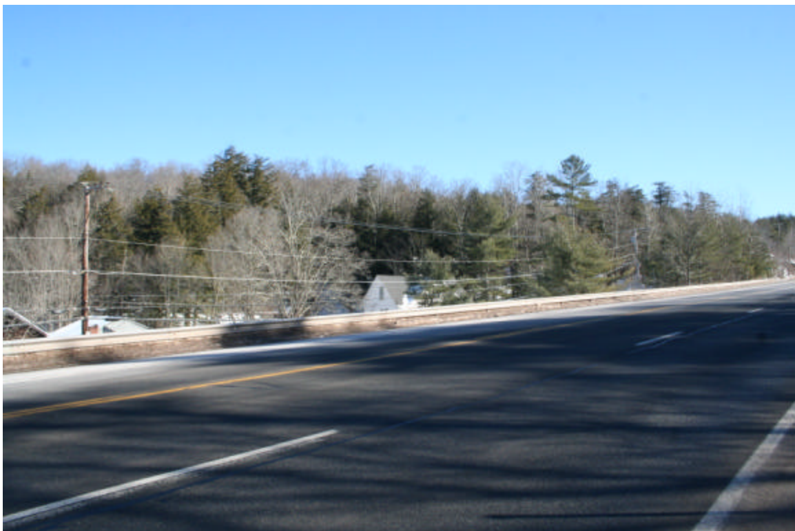
Photo 56. Portion of panoramic view from the west end of the proposed sewer main route, facing northwest.
