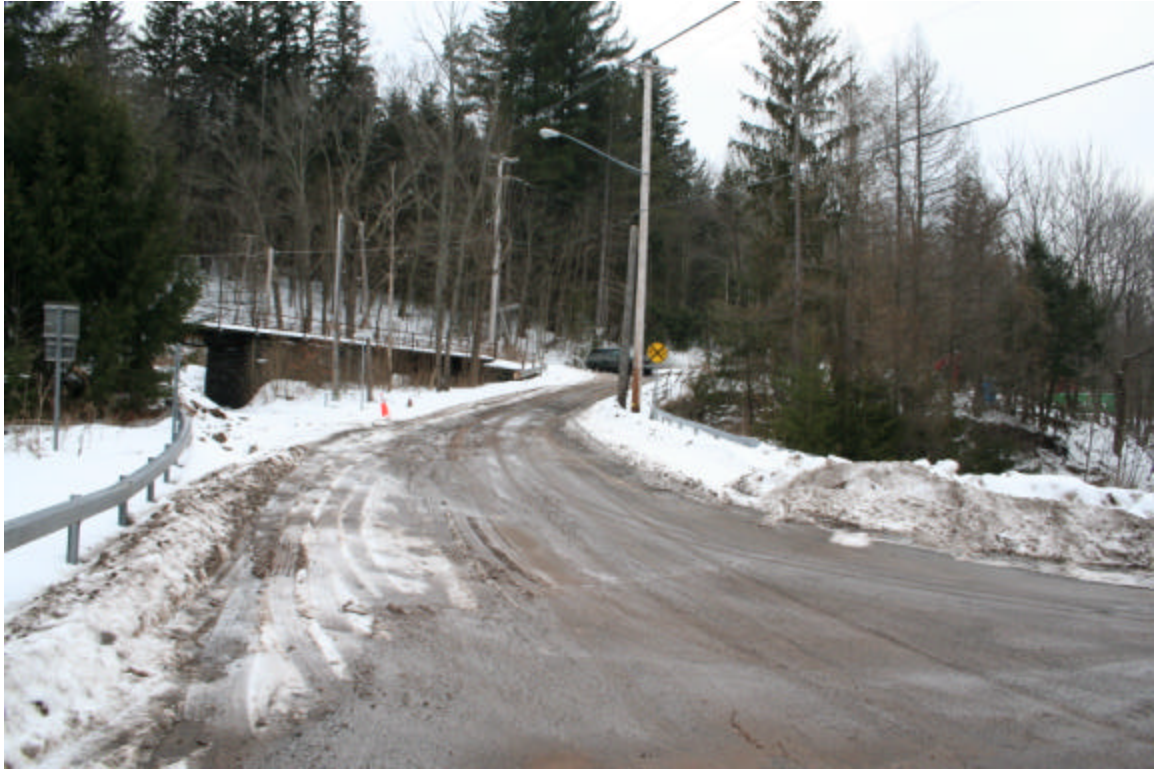
Photo 24. Portion of panoramic view from the intersection of Depot Street and NYS Route 28, facing southwest.
