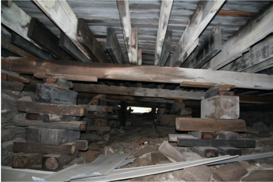
Photo 22. View of railroad ties supporting the floor of the depot, facing southeast.
