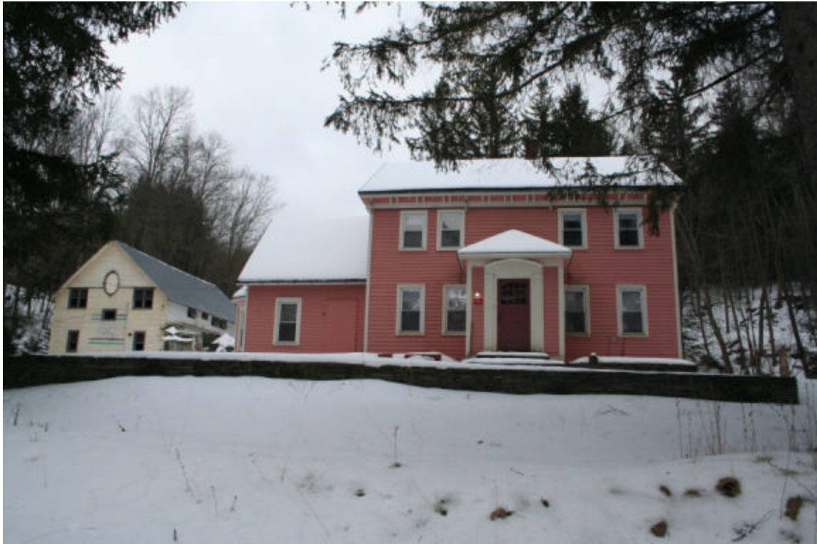
Photo 15. View historic structure on the south side of Depitts Lane, facing south.
