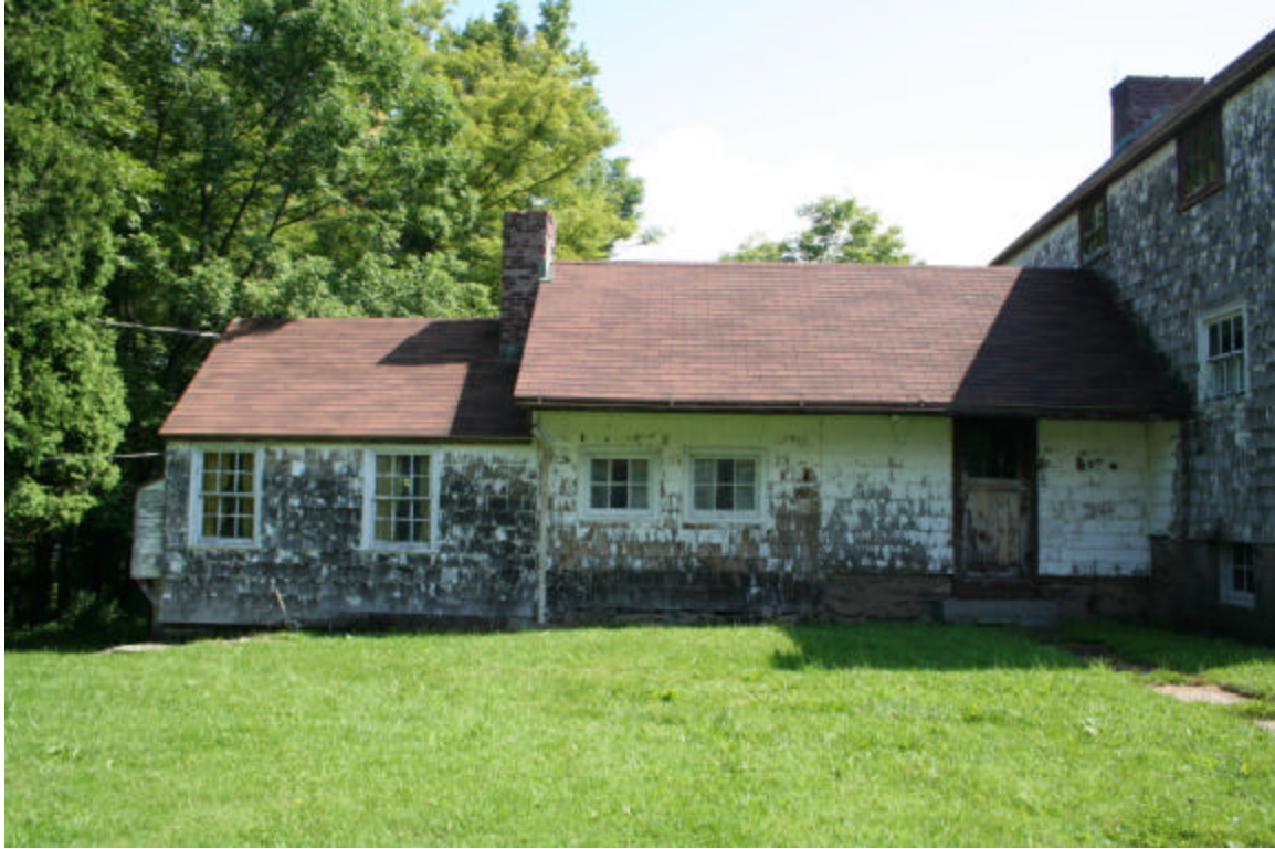
Photo 71. View of east façade of farm house on the north side of NYS Route 44A, facing east.
