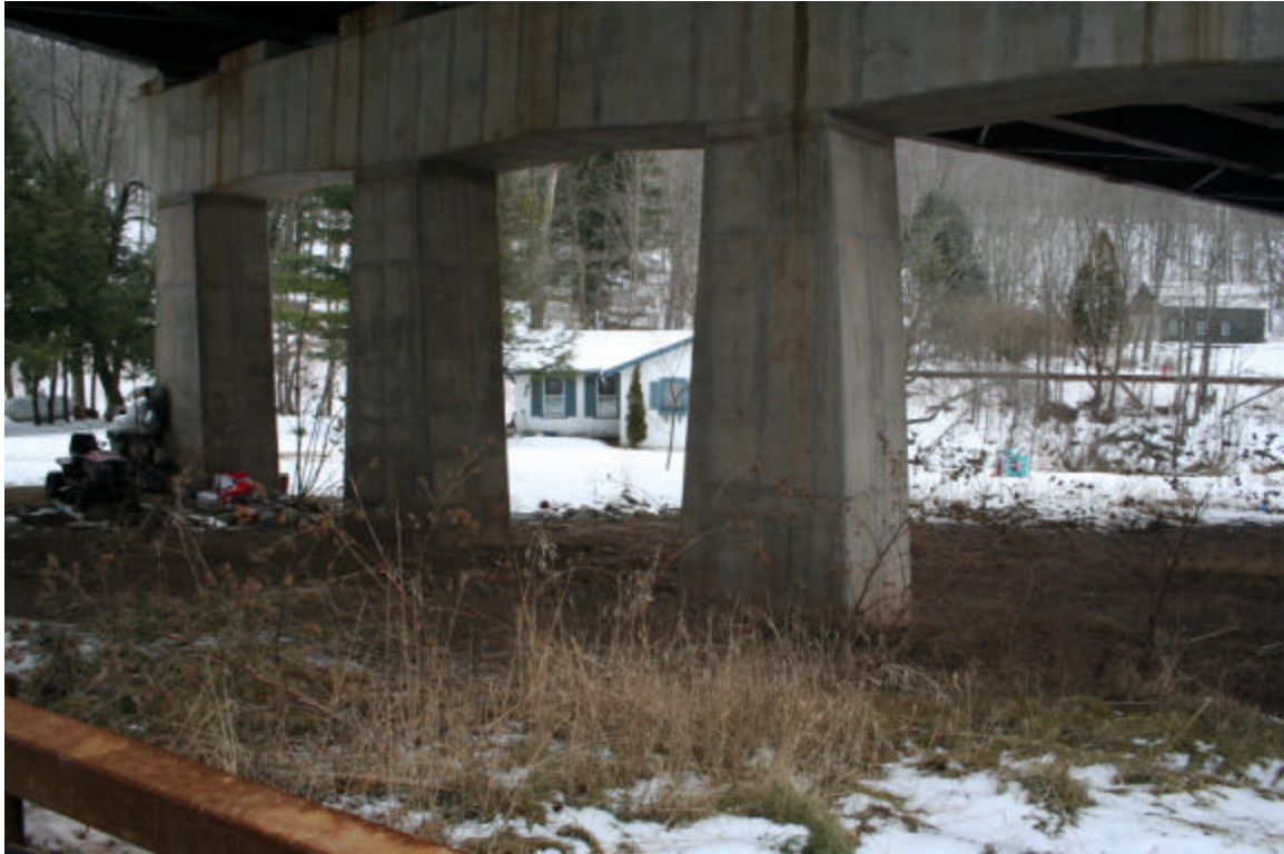
Photo 76. Portion of panoramic view from the east end of the proposed sewer main route, facing northeast.
