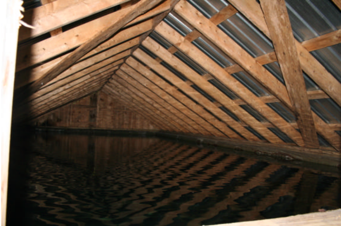
Photo 65. View of the interior of spring house in the northern part of the northern APE area, facing southeast.
