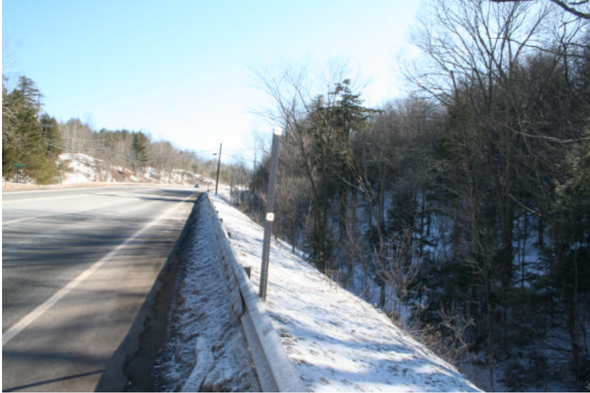
Photo 57. Portion of panoramic view from the west end of the proposed sewer main route, facing west.
