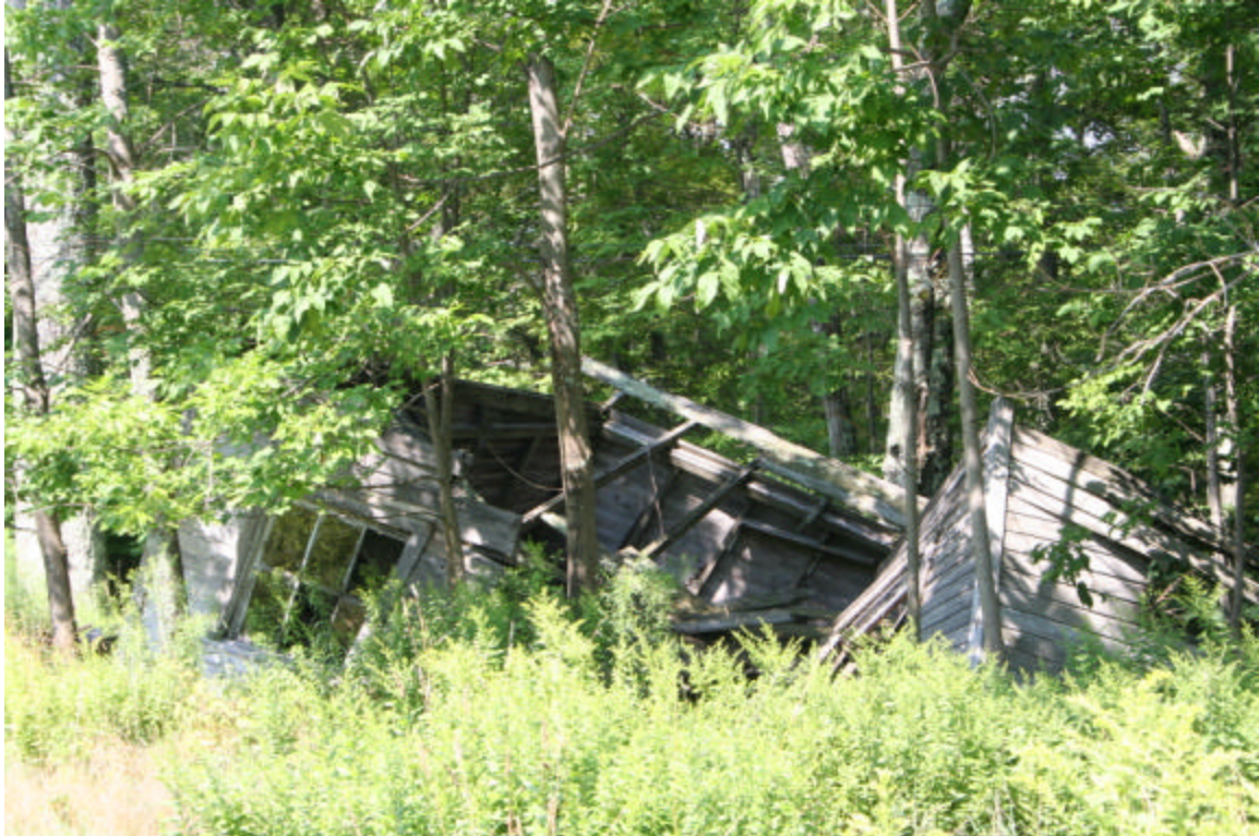
Photo 75. View of collapsed outbuilding at the farm complex on the north side of NYS Route 44A, facing north.
