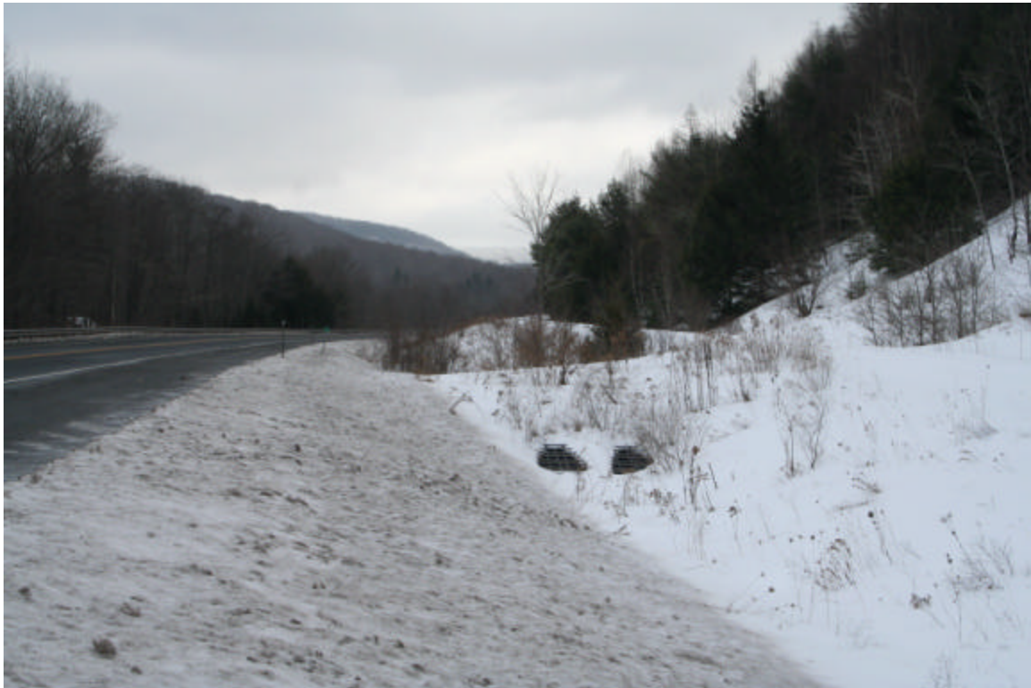
Photo 34. View of culvert along the proposed water main route on the south side of NYS Route 28, facing southeast.
