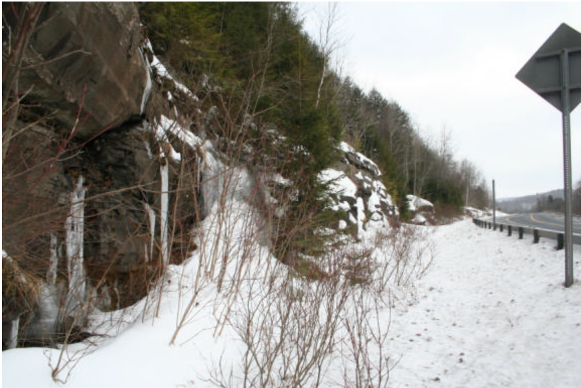
Photo 38. View of exposed rock cuts along the water main route along NYS Route 28, facing northwest.
