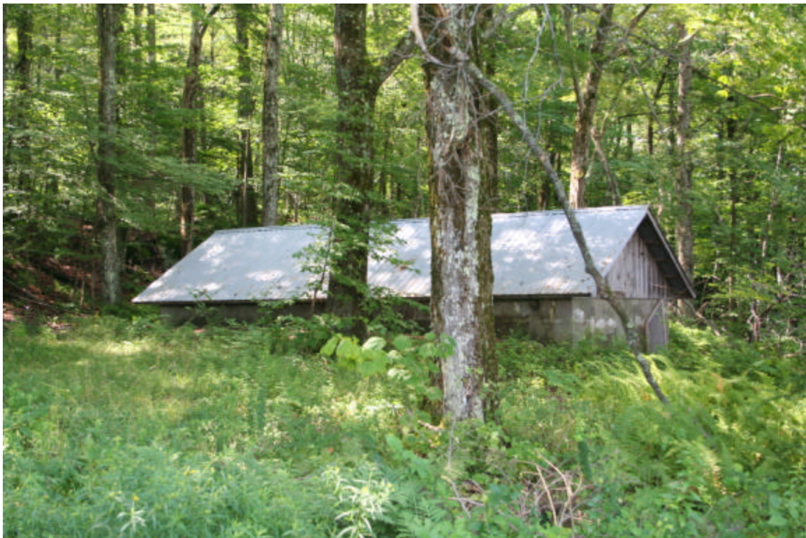
Photo 64. View of spring house in the northern part of the northern APE area, facing southwest.
