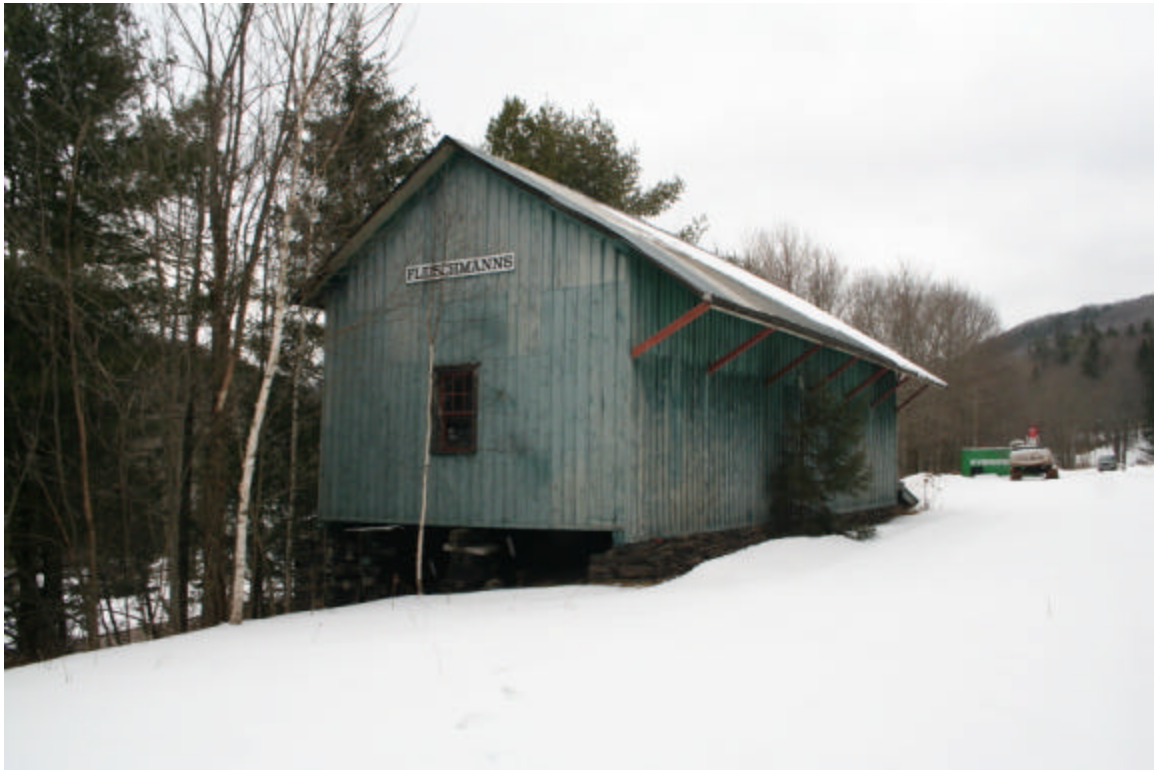
Photo 20. View of Fleischmanns railroad depot, facing northeast.
