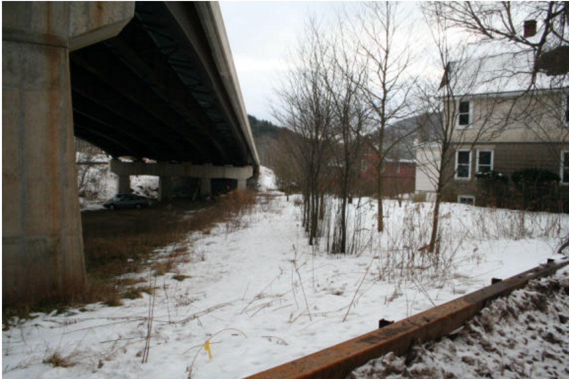
Photo 77. Portion of panoramic view from the east end of the proposed sewer main route, facing southeast.
