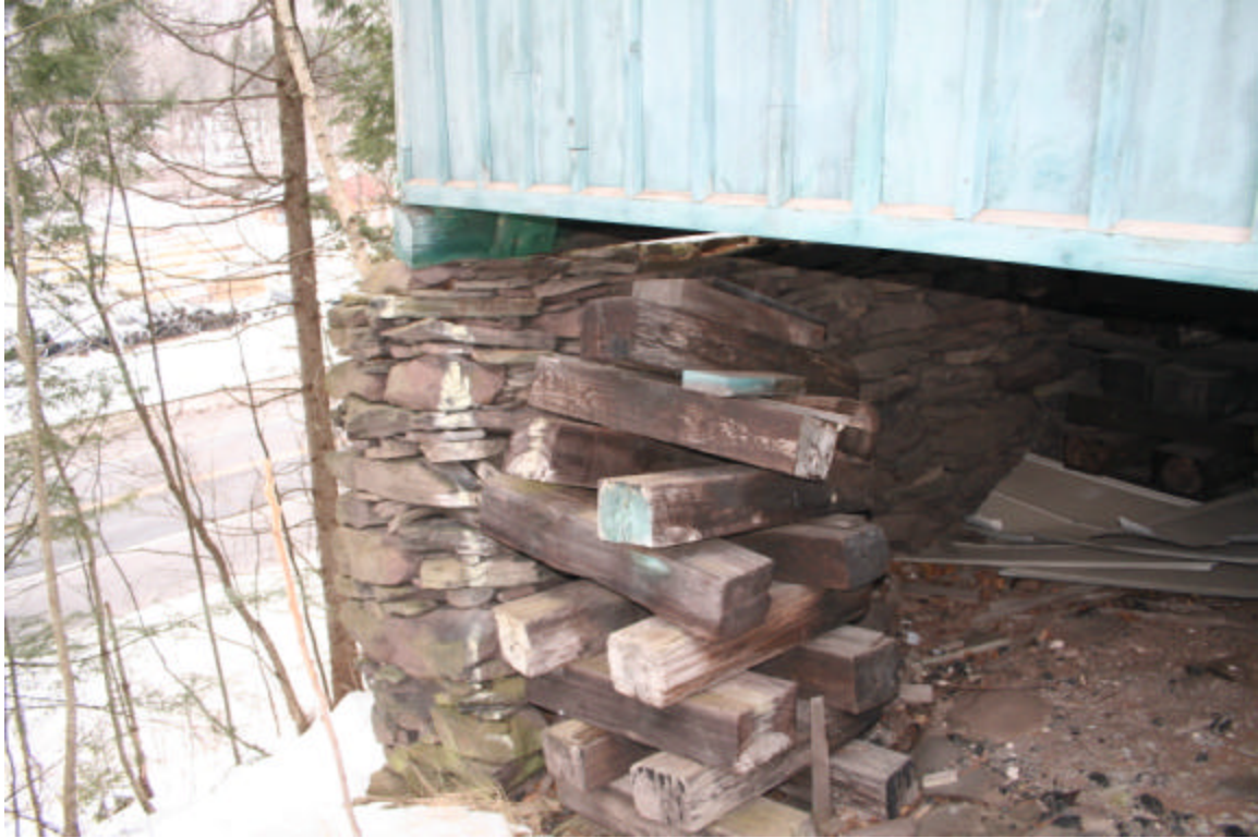
Photo 21. View of collapsing sill on the northwest corner of the Fleischmanns railroad depot, facing east.
