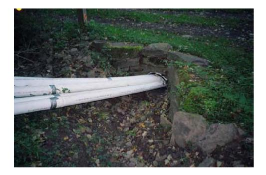
**Photograph 2:** Water from K2, K3 and K4 is carried downhill through six platic pipes (two per well) and discharged into a steel culvert under a driveway.
