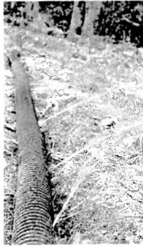
A biofiltration system 150 feet long can disperse up to 200 gallons per minute — nearly 300,000 gallons per day.
