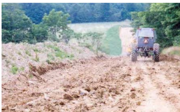
Fig. 1. A typical deep ripping phase of this practice, during the first in a series of progressively deeper “rips” through severely compressed subsoil.
